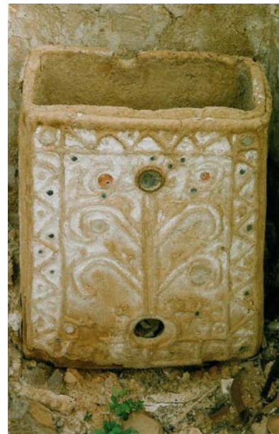
Building Construction. Fig. 19 Grain storage made of fiber-reinforced mud (Kutch, Gujarat, India) (photo by the author).
